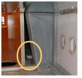
Tube lines placed on a tray Above the air ducts (preferred solution)
